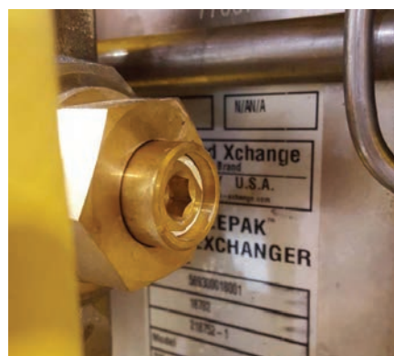
V3 INDICATOR OPEN POSITION
