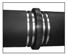
ALIGNMENT— After aligning the two pipe ends, pull the gasket into position, centering it between the grooves on each pipe. The gasket lip should not engage with either of the pipe grooves.
