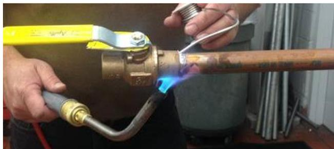
Figure 2 – Heat valve cup area and apply solder
